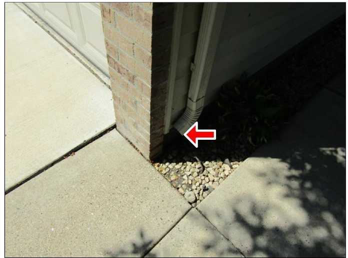
One example. A majority of the downspouts lack proper extensions
