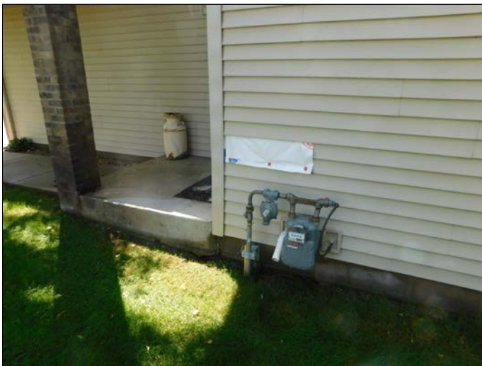
(5) There were loose, damaged or missing pieces of vinyl siding at the building. Have the loose pieces of siding secured to lower the potential for water intrusion or wind damage.
