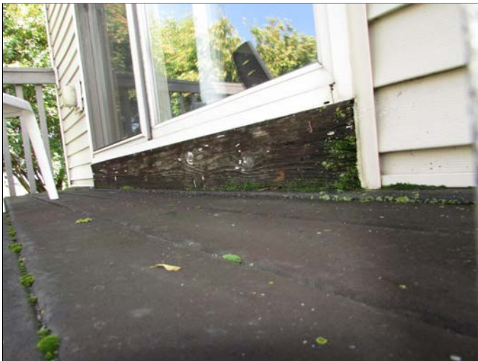
Typical type of deterioration where water splashes off decks without gutter protection
