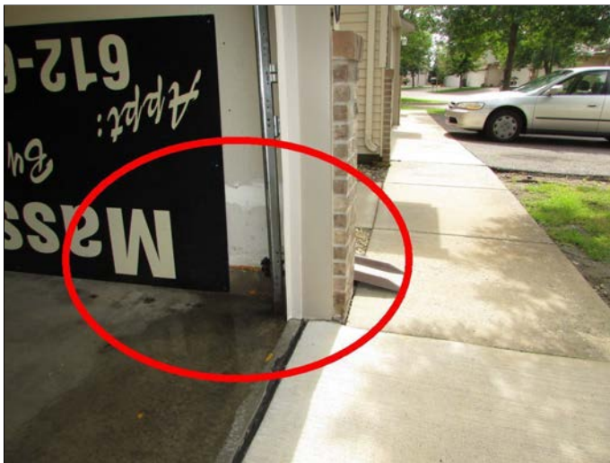
Moisture noted at inside of garage at unit 9163
