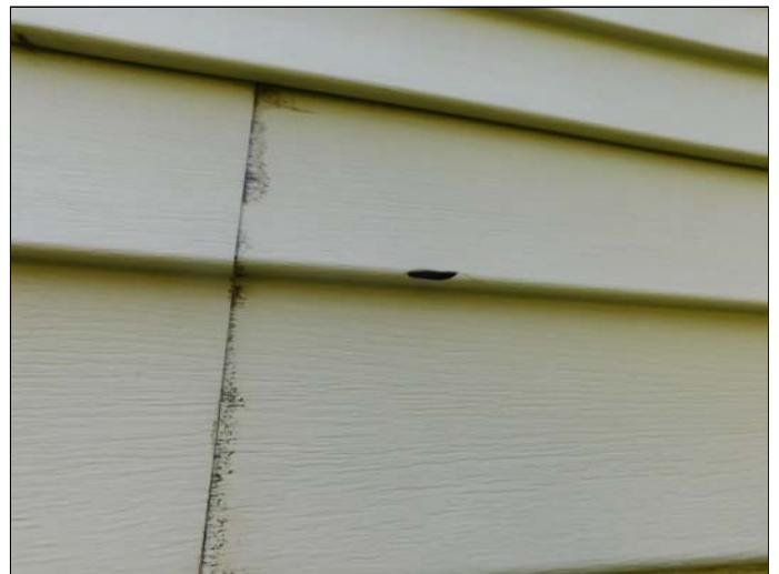
(5) There were loose, damaged or missing pieces of vinyl siding at the building. Have the loose pieces of siding secured to lower the potential for water intrusion or wind damage.
