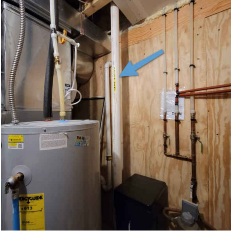
radon pipe in utility room
