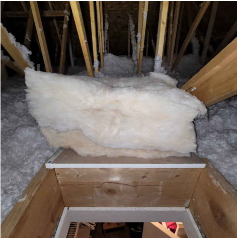
fiberglass batts at access panel
