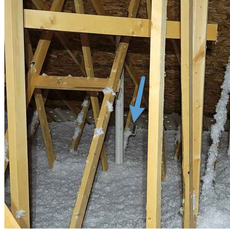
radon pipe and outlet in attic
