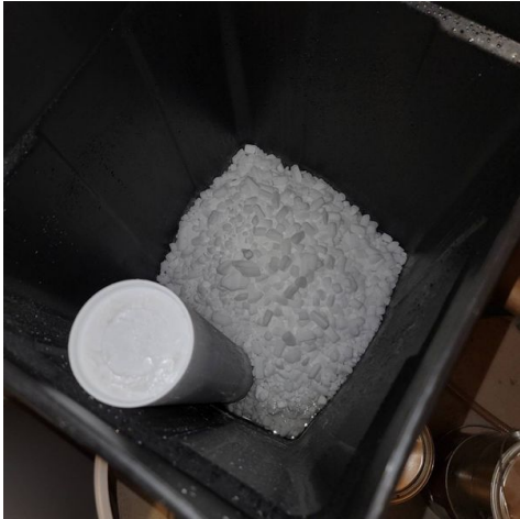
salt in storage tank
