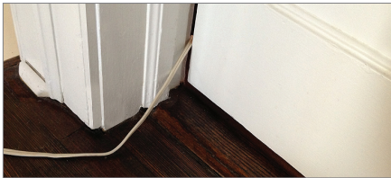
At loose electrical connections or cords damaged by doors closing on them
