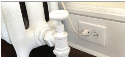
Through wires or cords damaged by heat, sunlight or humidity
